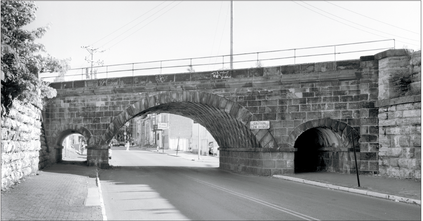
Reading built this stone bridge in Reading, Pa., in 1857, and it's still in use by Norfolk Southern. All three arches are skewed—the railroad crosses the street at an angle—uncommon for stone bridges. Jet Lowe, Historic American Engineering Record
