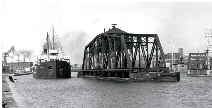
A ship passes a Canadian National double-track Warren swing bridge (with the operator's shack in the middle) in the 1930s. Swing spans provide a clear channel, but can be a navigation hazard because of their position in the waterway. Canadian National
